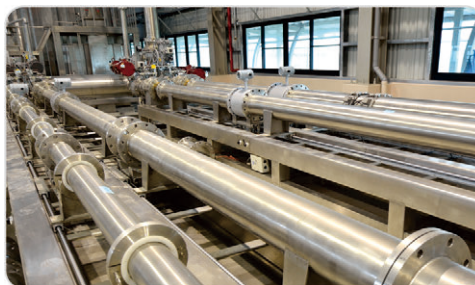
Piping system II (Maximum diameter is 300mm)
